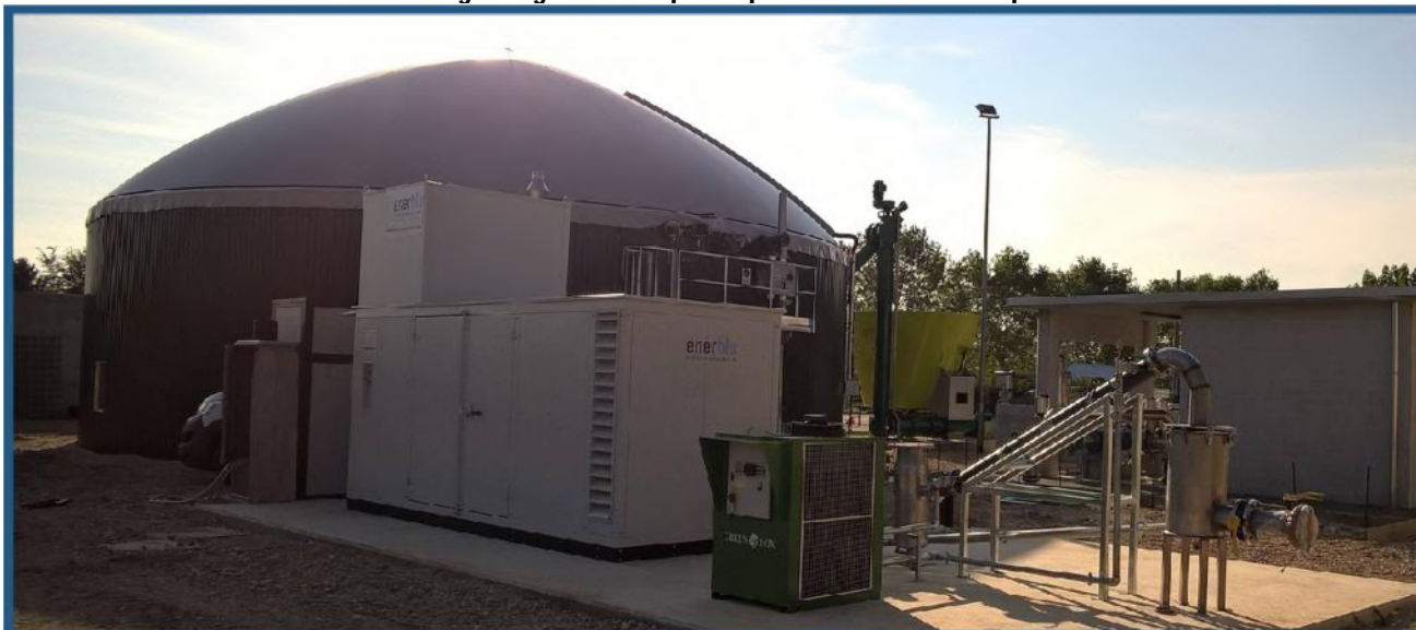
REC2 100 BIOGAS biogas cogeneration powerplant with an electric power of 100 kW e
