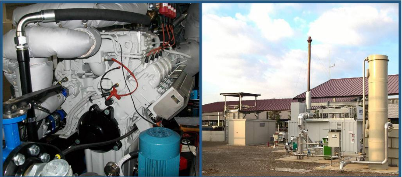
REC2 250 BIOGAS biogas cogeneration powerplant with an electric power of 250 kW e
